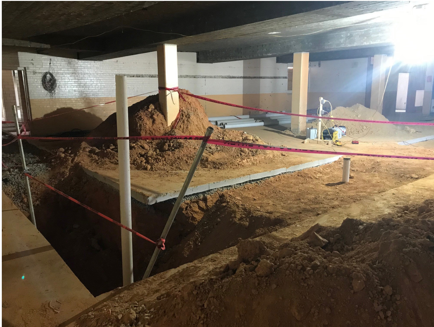
Demolition underway - New Sewer service partially installed
