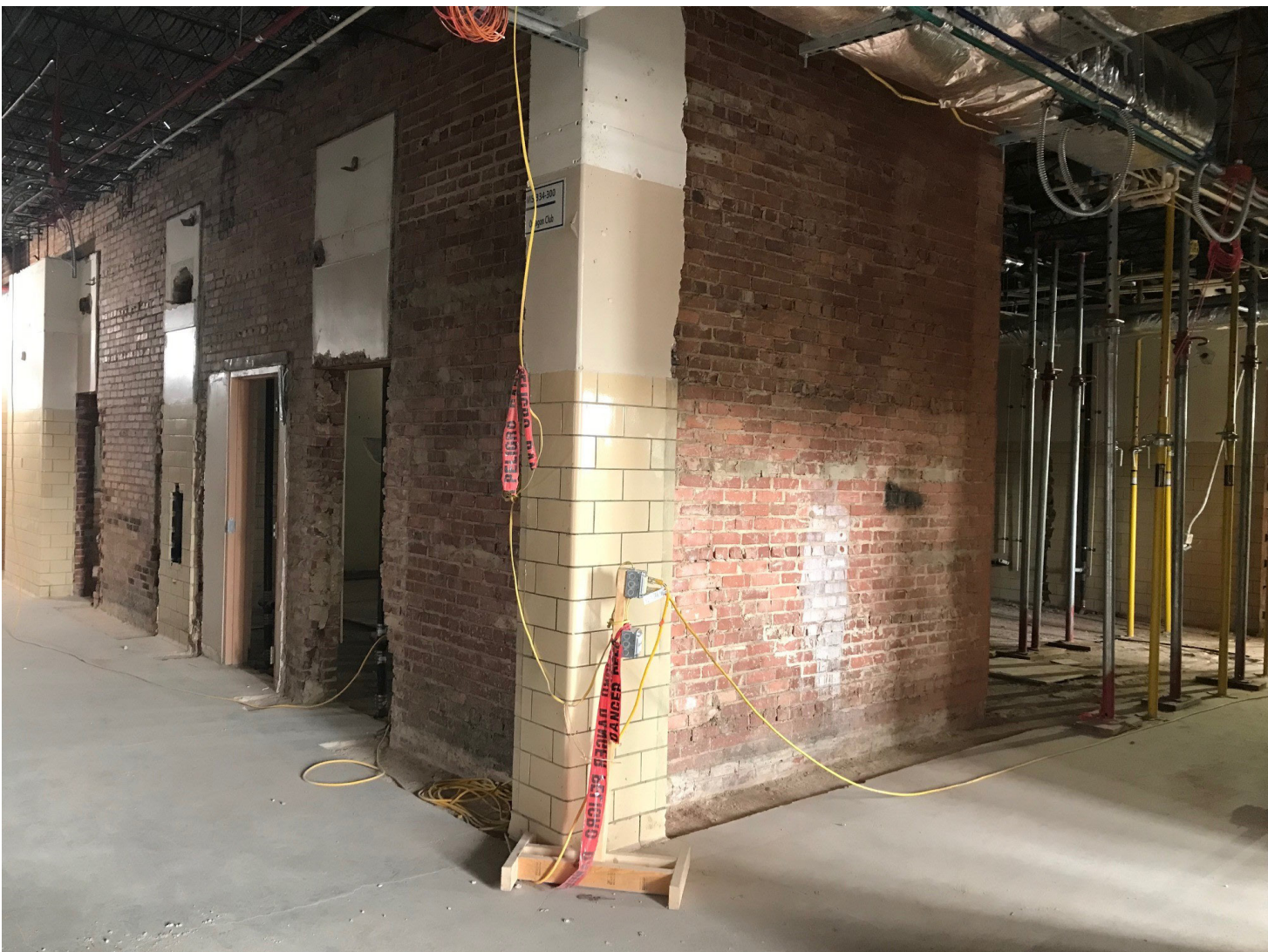
2nd Floor Demolition approximately 100% complete - Note structural shoring
