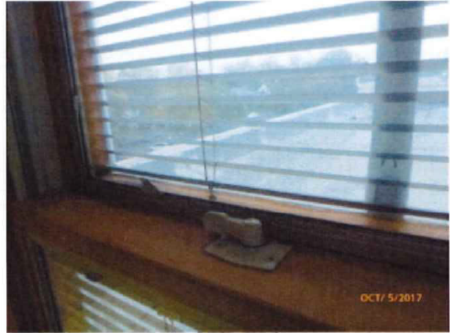
Interior of windows
