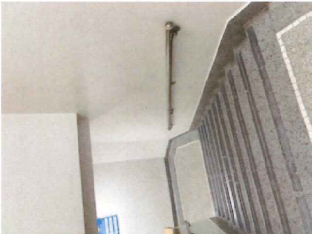
Non-compliant handrails
