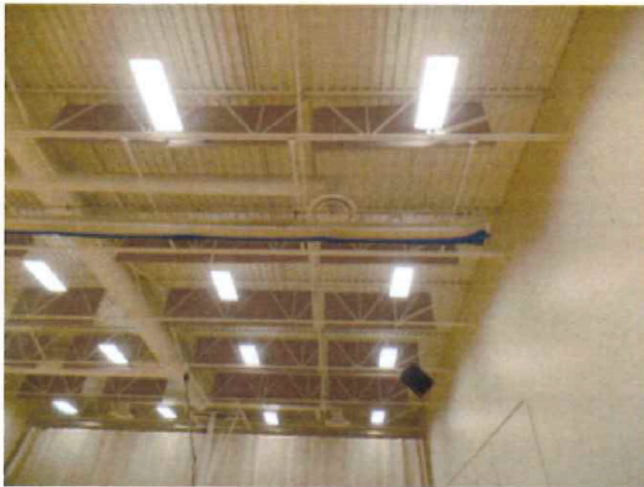
Metal roof deck
