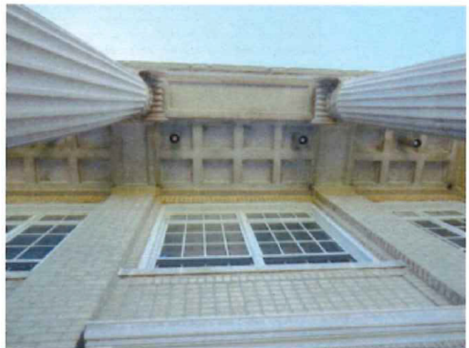
Cast in place concrete at roof level
