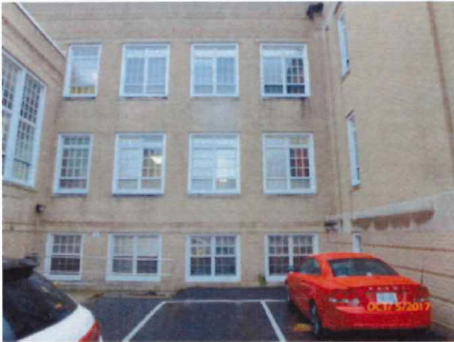
Exterior aluminum clad windows
