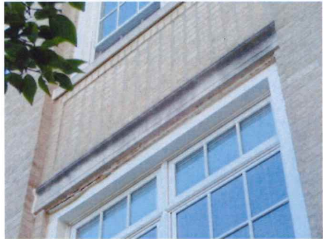
Add weeps at lintels and sills
