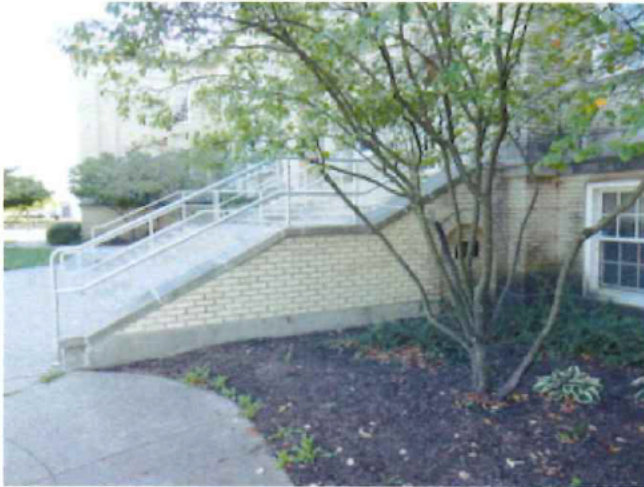
foundation wall at steps
