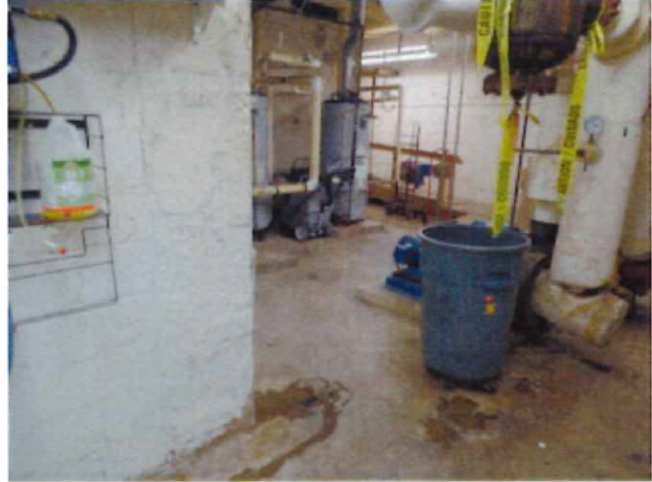
Test for lead paint
