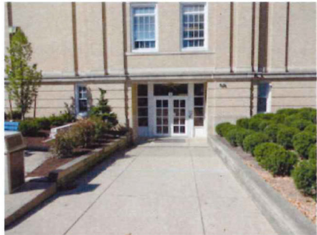
ADA compliant ramp and entrance
