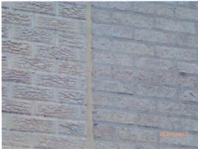
Re-caulk expansion joints
