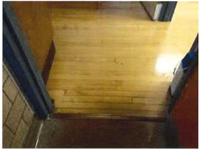
Wood floors in classrooms
