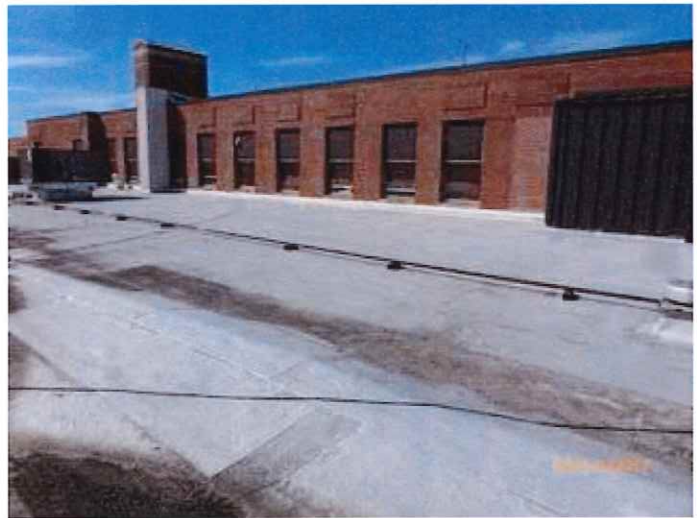
Replace lintels on 3rd level
