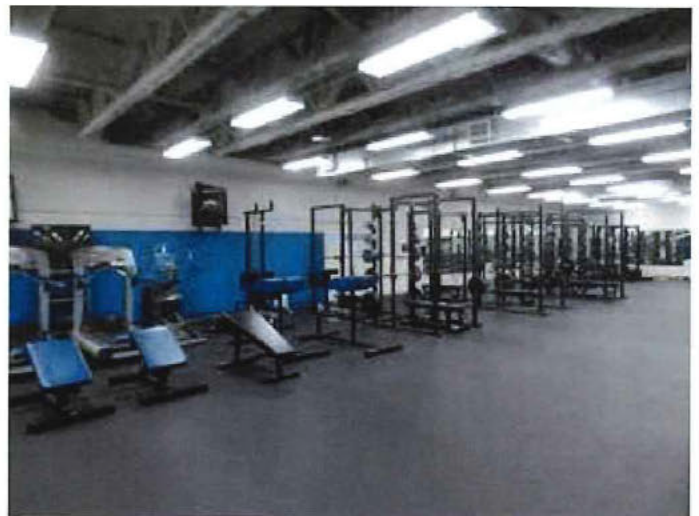
Steel bar joist with spray on fire proofing
