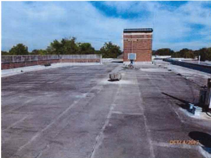
Built up roofing
