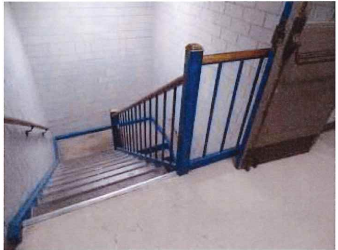
Non-compliant handrails
