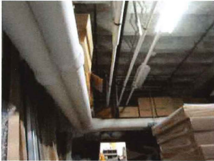
Precast concrete deck
