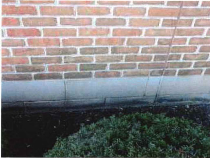
Foundation wall exposed
