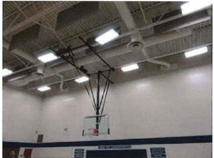
Exposed metal deck
