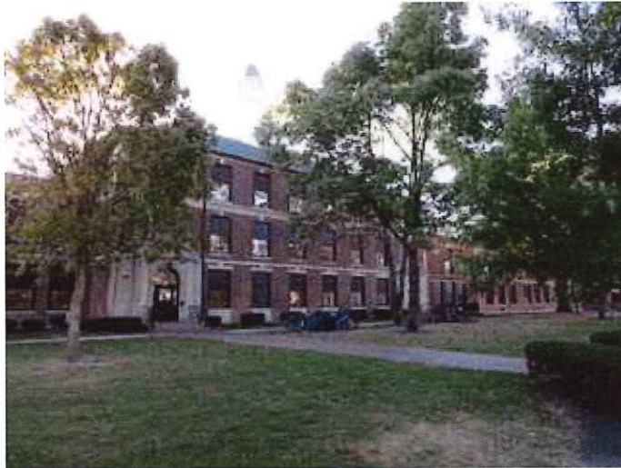
Brick building cleaned and sealed
