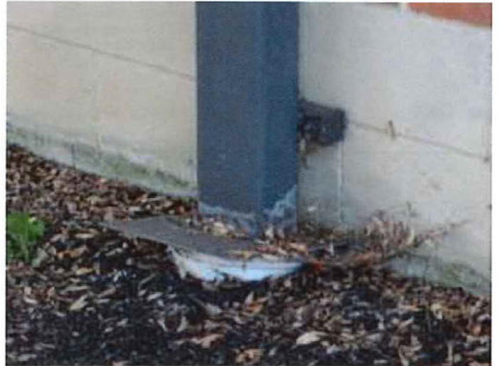
Foundation wall at downspout
