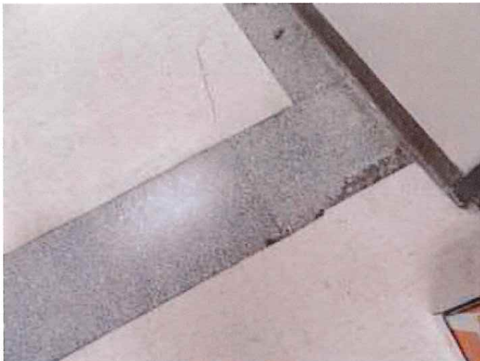
Terrazzo and VCT flooring
