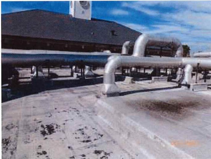
Built up roofing
