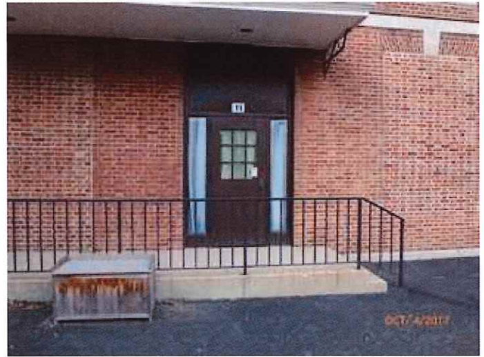
Exterior steel door and frame
