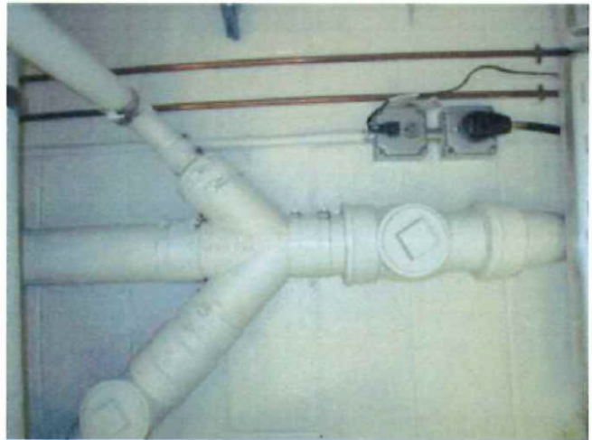
Exposed Sanitary Stack
