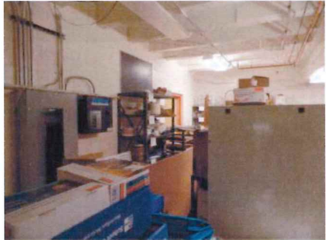
Cast in place concrete floor deck
