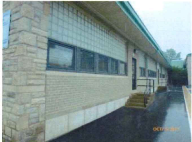
foundation wall exposed
