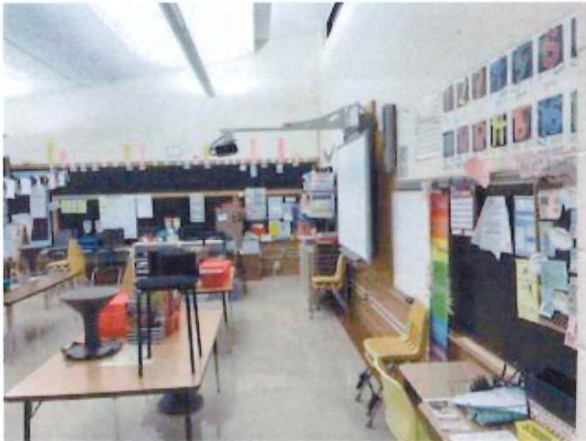
Joists enclosed by acoustical ceiling
