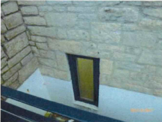
Foundation wall exposed
