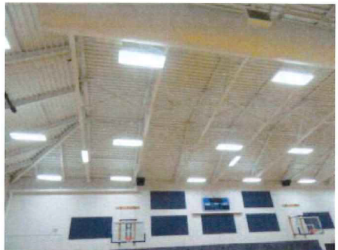
Exposed metal deck
