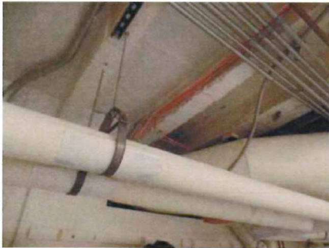
Cast concrete deck
