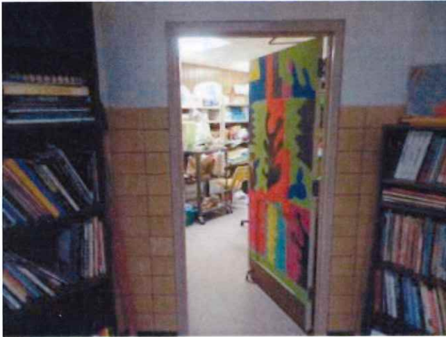
Asbestos containing floor tile
