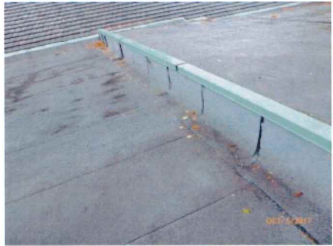
Metal cap flashing
