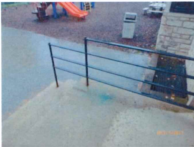
Non-compliant handrails
