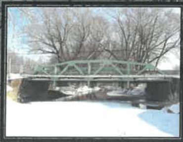
Cover photo: Completed bridge P-301 on Campbell Street in Perkins Township. Inset photo: P-301 prior to construction.
