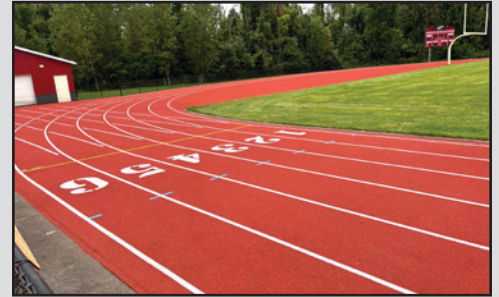
Track After Resurfacing
