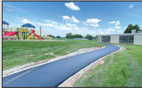
New Playground Path Installed
