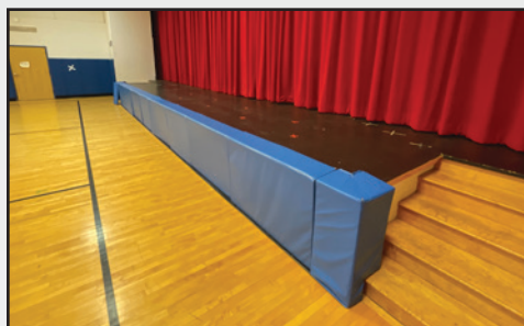
Primary Gym Stage Before
