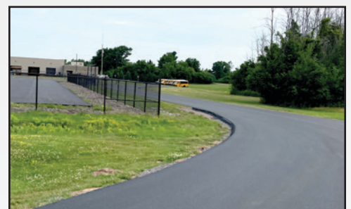
Paved Hawk Drive After
