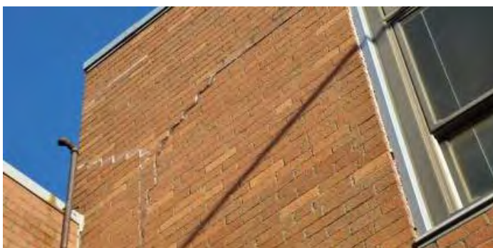
Left & Bottom: Masonry settlement at original building Top: Roof repair needed at library/media center
