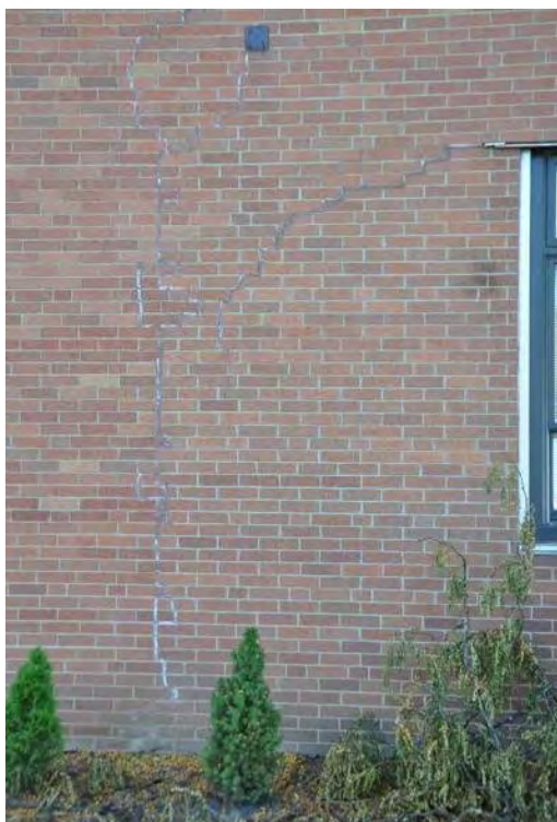
Left & Bottom: Masonry settlement at original building Top: Roof repair needed at library/media center
