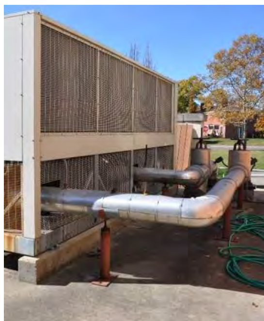
Air Cooled Chiller replacement
