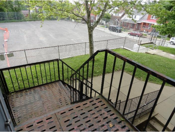
Emergency Exit Stairs leading to play area.
