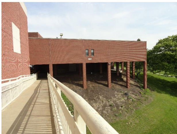
Exterior at the rear of the building.
