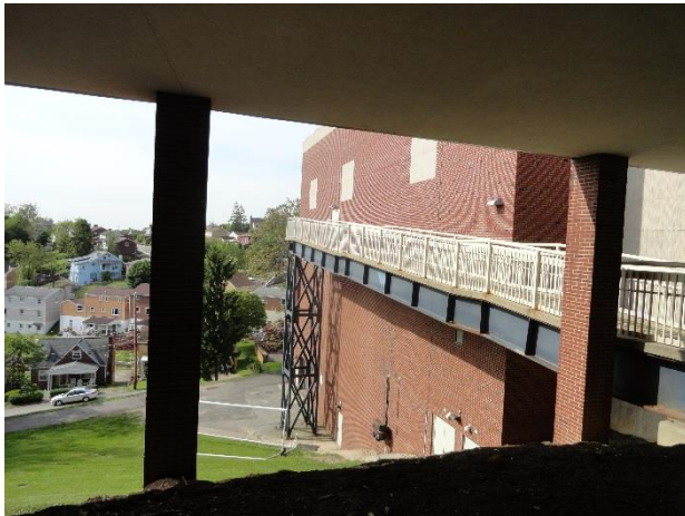
Emergency exit ramp from gym area.
