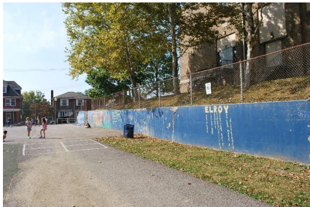
Retaining wall located between building and playground.
