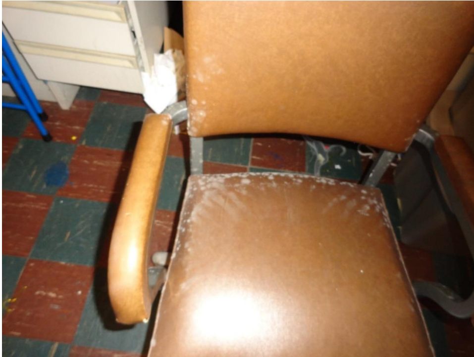
Lower Level mold-like substance on surfaces.
