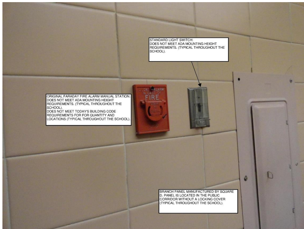
Original Faraday fire alarm, standard light switch and branch panel do not meet today's code requirements.
